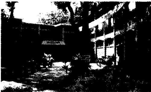
Front View of the Library
