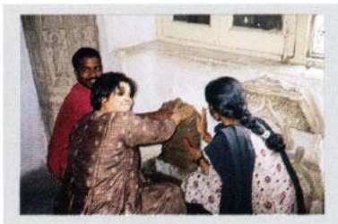
Affected Limestone Sculpture in the Amaravati Gallery is being Pouliticed with Paper Pulp
