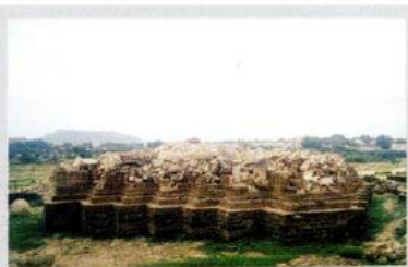
Rao Lakha Chattri ( 18th Century A.D.), Bhuj after Earthquake
