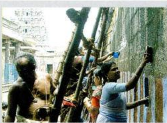
Officials are Chemically Cleaning Moss and Lichen Affected Temple Compound Wall
