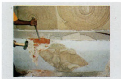
The Wall is being Scooped out for Removing a Limestone Sculpture
