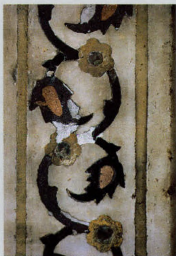
Plaster In-fills Destroy the Effect of the Contrast between Marble and Semi-precious Stone, Which is Seen to Better Effect in Those Areas Which Still Retain Their Inlay.
