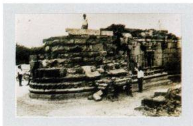
Frontal Mantapa of Amman Shrine, Pushpavaneswara Temple, Puvallakudi, Pudukkottai Dsistrict before Structural
