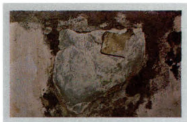
Embedded Limestone Sculpture after Extraction of the Salts
