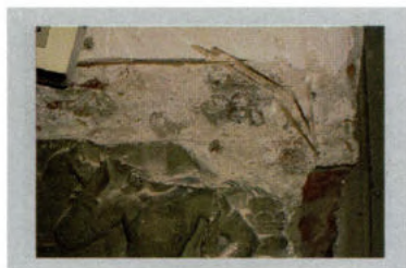
The Wall is being Marked for Scooping the Wall
