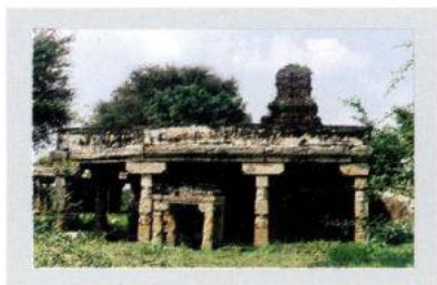
Conservation of Soundararajaperumal Temple, Irumbanadu, Pudukkottai District before Structural Conservation
