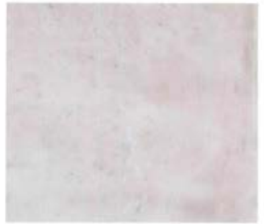
Wall after conservation using Moghul plaster
