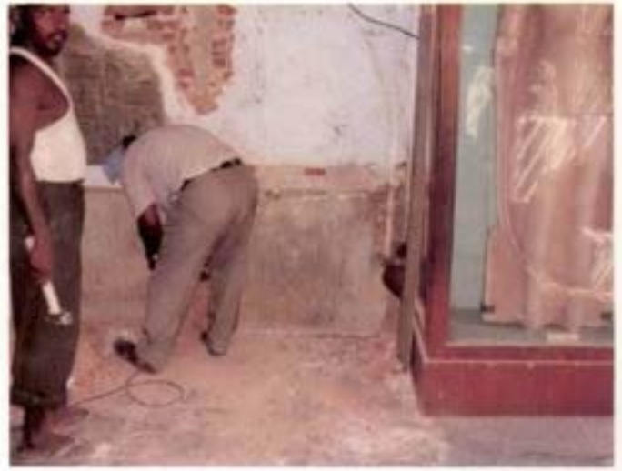
Removal of embedded Amaravati Sculpture from the walls using power tools.
