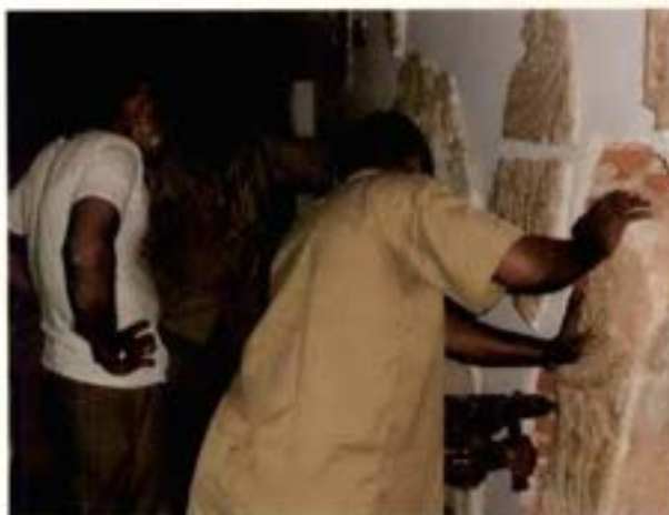
Removal of embedded Amaravati Sculpture from the walls using power tools.
