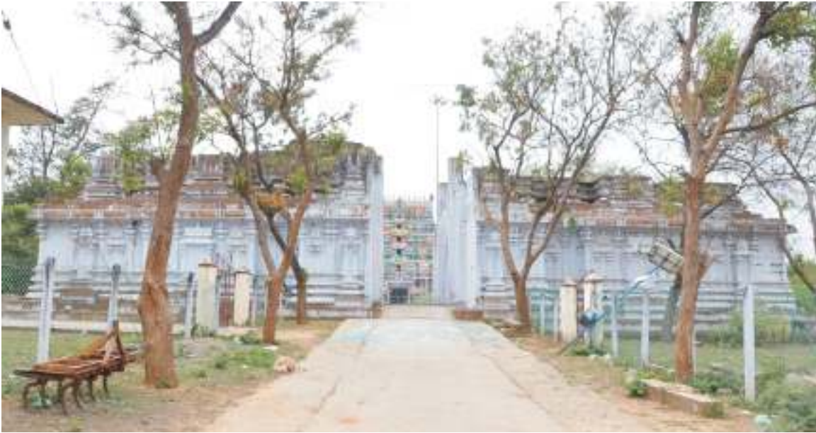
Front view of the entrance
