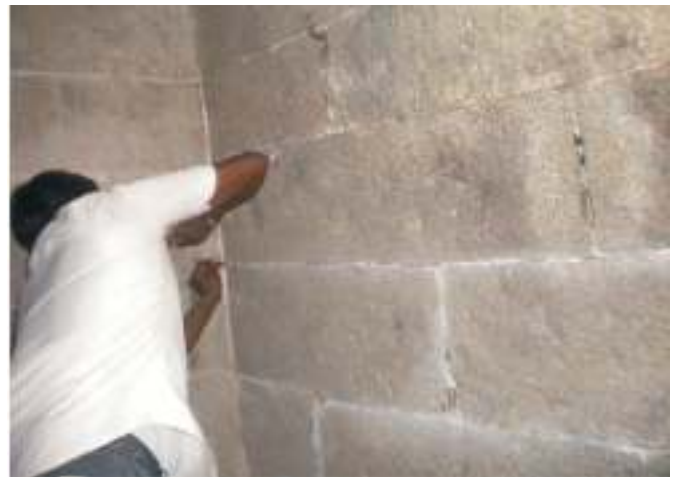
Filling holes with mixed lime mortar
