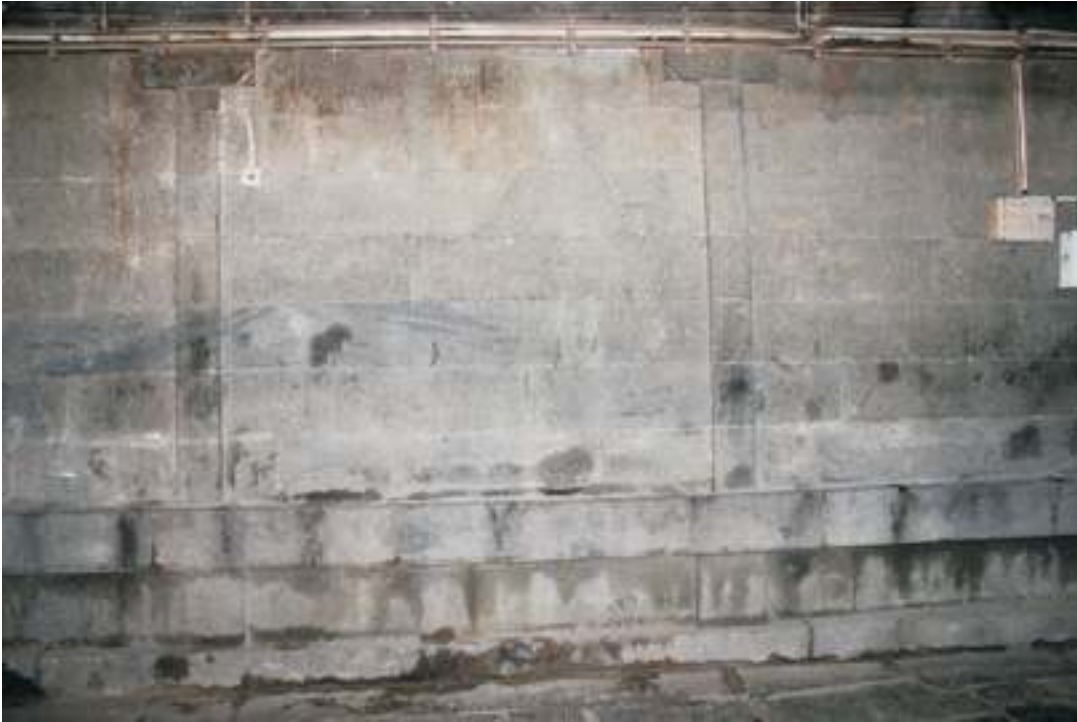
North wall of Madappalli
