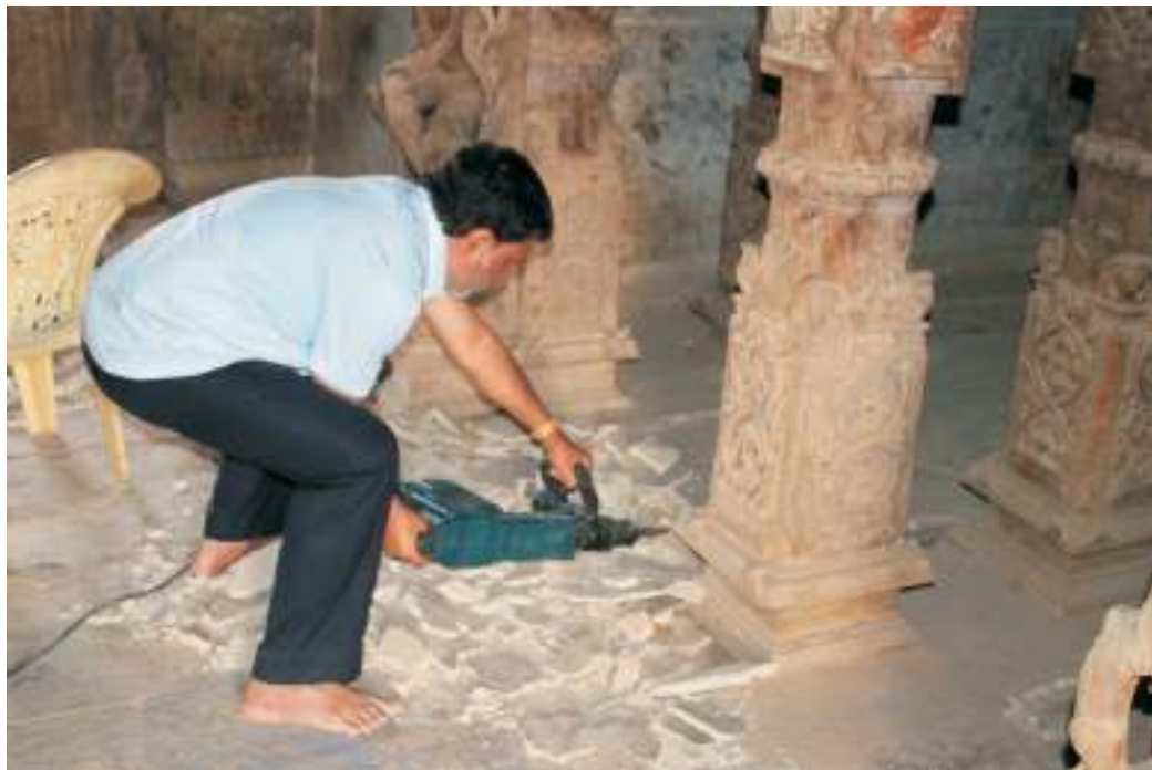
Use of Power tools for removing old cement flooring.
