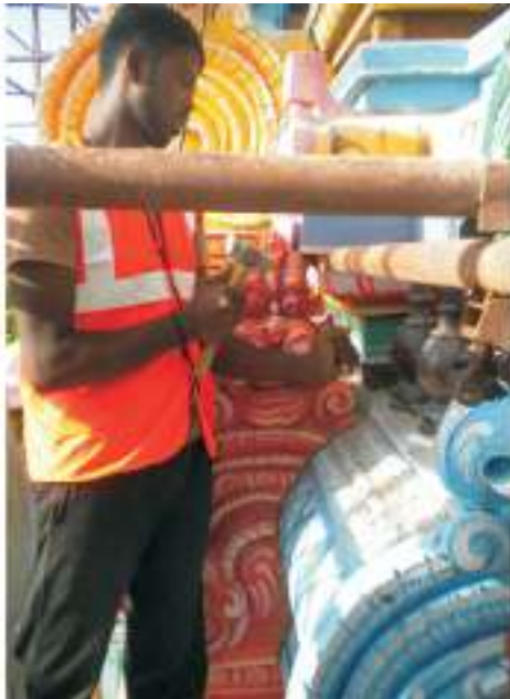
During application of Ground Lime Mortar Mix twice with time interval
