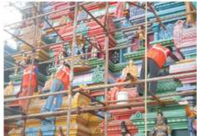
During application of Ground Lime Mortar Mix twice with time interval
