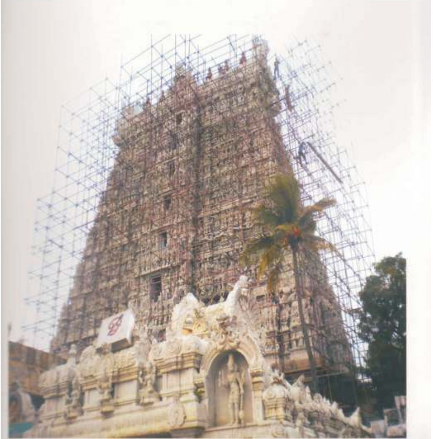
Scaffolding for water tightening - Suchindram
