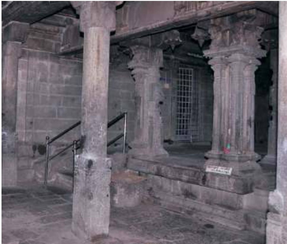
East wall of Mahamandapa of Narumpoonathaswami temple
