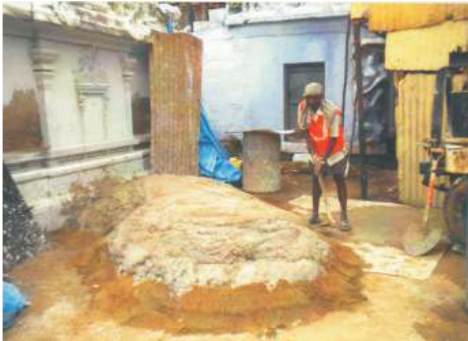
Lime Mortar Mix under preparation
