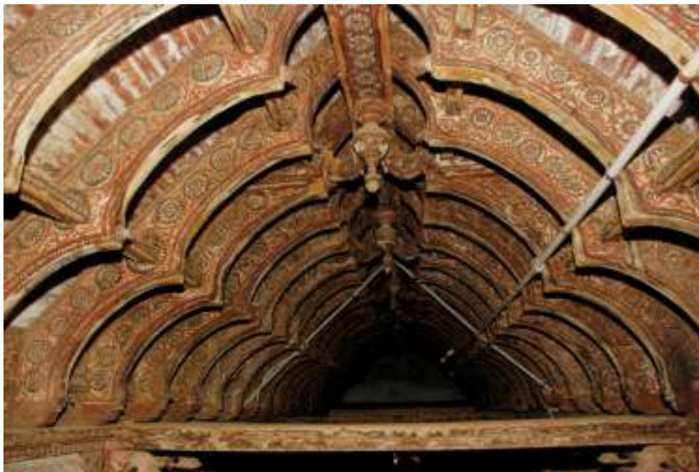
Sala roof - closer view
