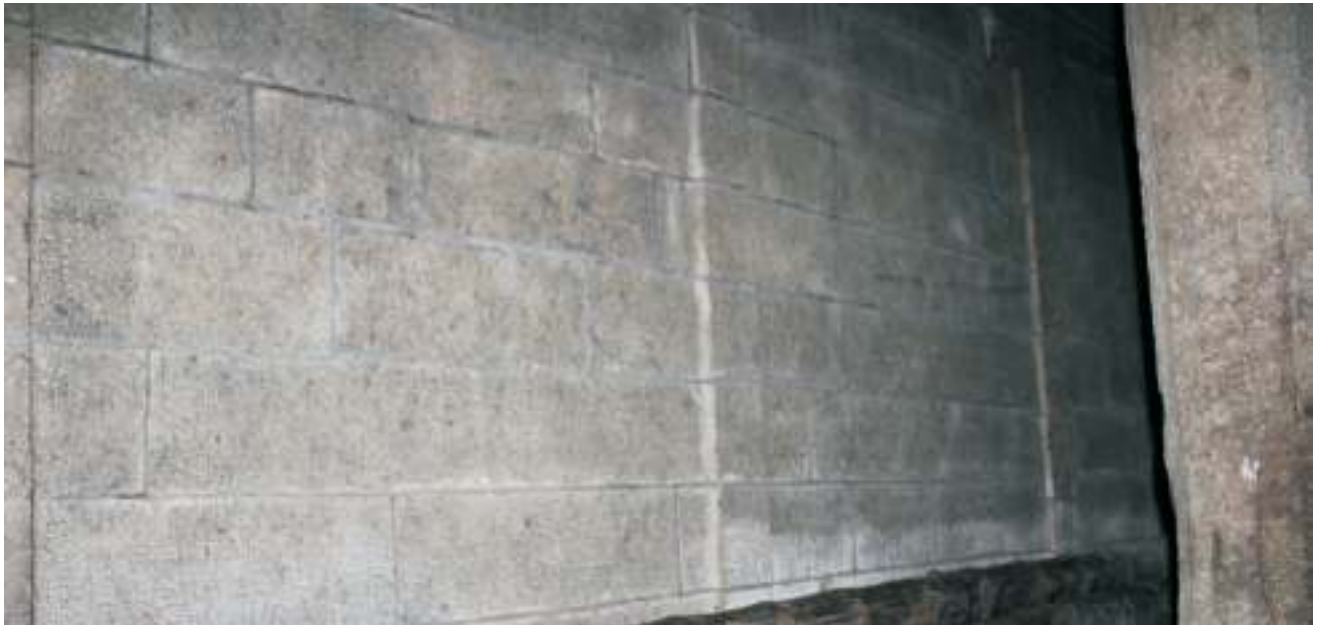
North wall of Mahamandapa of the Narumponathaswami temple
