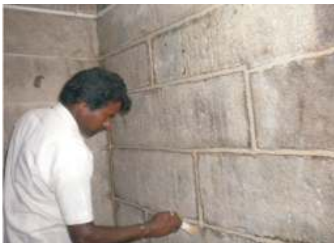
Finished with Sbbara lime mortar mix ( Moghul polish)
