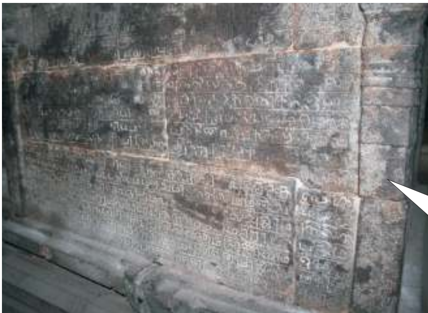
East and North wall of Chandikesvara shrine
